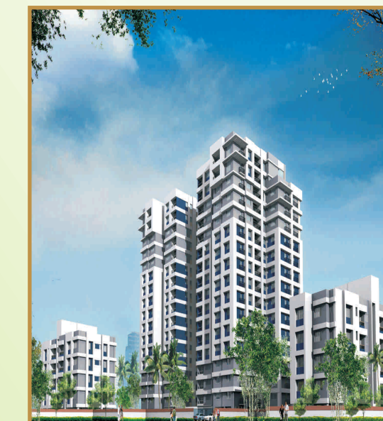
Rohra Heights, G+16 hi-rise at New Town
